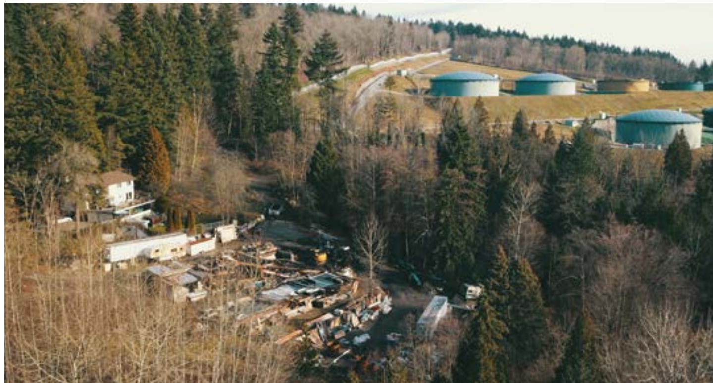
In January 2019, a fire burned down a private building (seen at left) just steps away from the Burnaby Tank Farm. Photo: Stand.earth
