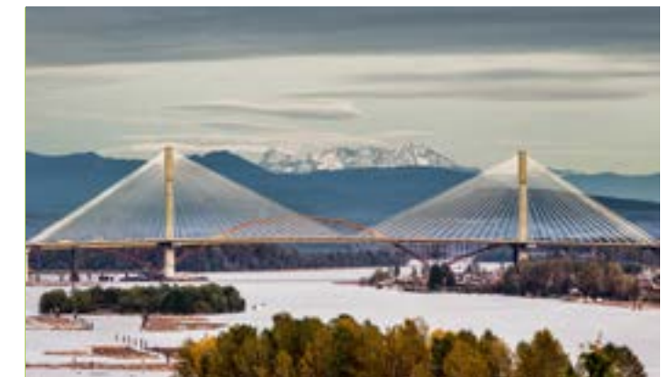
Trans Mountain plans for the pipeline to cross the Fraser River just east of the Port Mann Bridge (seen above). Photo: Jason Drury, Creative Commons
