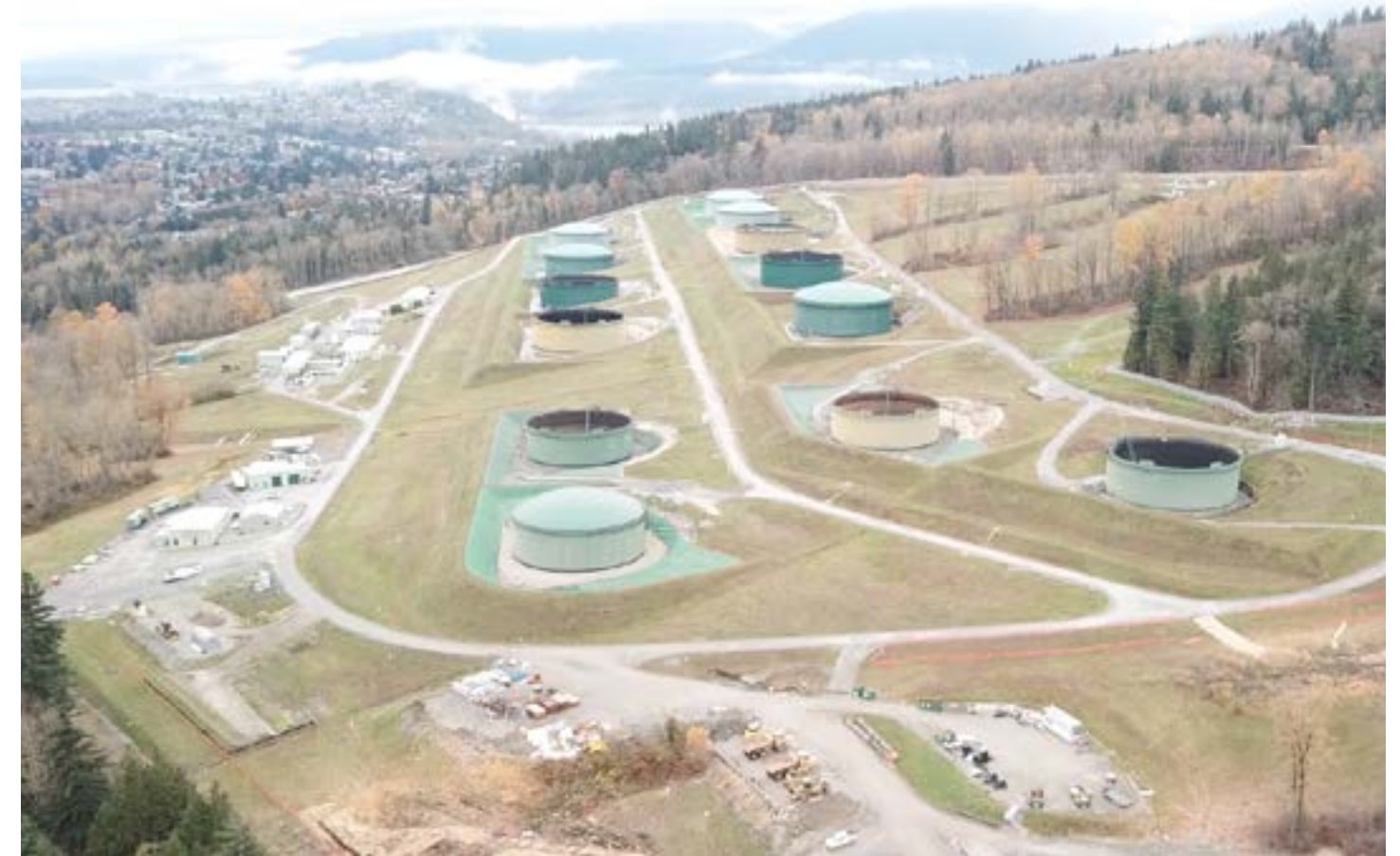
Several oil storage tanks at the Burnaby Tank Farm employ floating roofs, which in an earthquake region can be a more dangerous alternative to fixed roofs. Photo: Stand.earth
