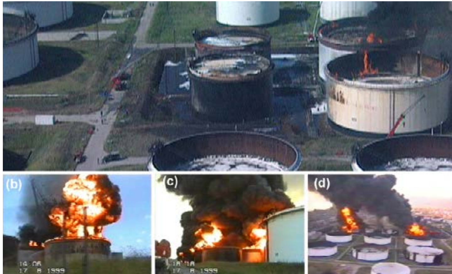
An earthquake in Turkey in 1999 caused damage to an oil refinery's floating roof tanks, which have a similar design to several oil storage tanks at the Burnaby Tank Farm. Photo: ResearchGate
